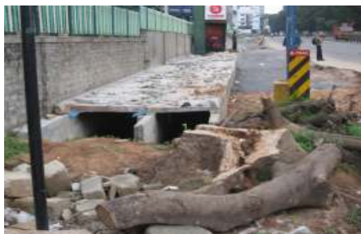
Concrete channels on widened Road
