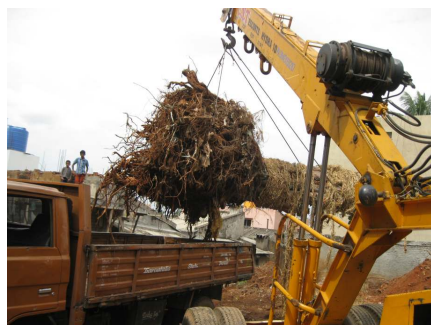
Uprooted tree being loaded on to the truck
